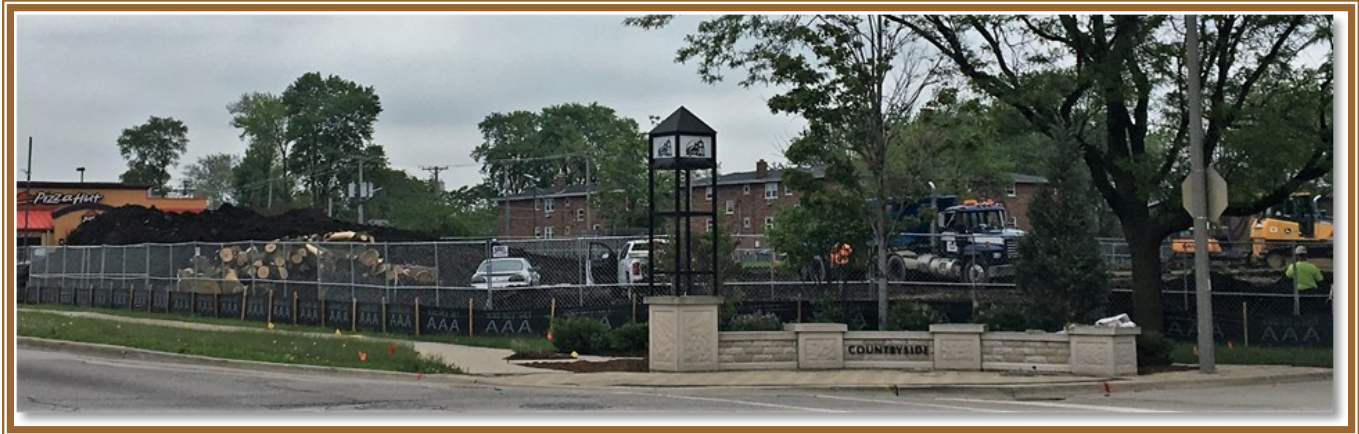
The site work began this spring at 5631 S. La Grange Road. Construction is expected to go through the end of the year.
